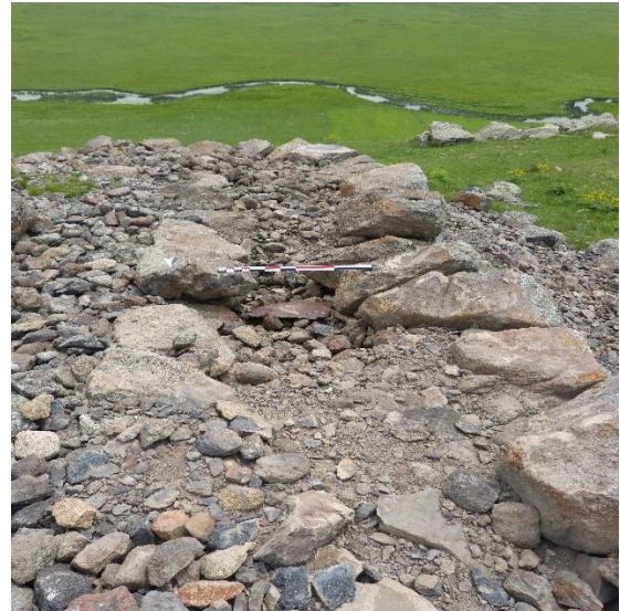
Fig. 12. The west wall of the western tower of Bellitepe.
