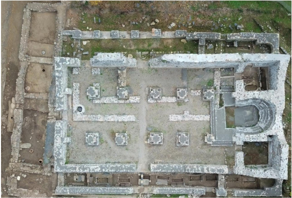
Fig. 22. Duruji Basilica, zenithal view.
